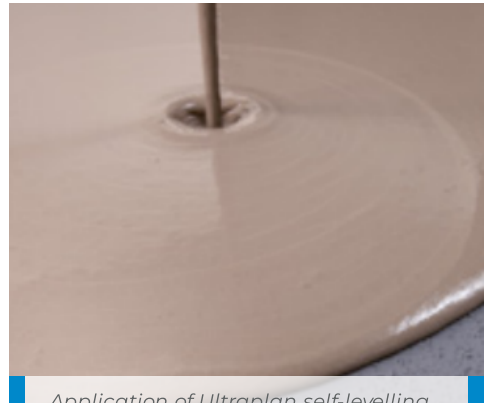
Application of Ultraplan self-levelling smoothing compound on dry Eco Prim Grip on old floor
