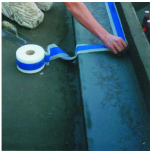
An example of Mapeband waterproofing a corner between the bottom and a side of a bath tub
