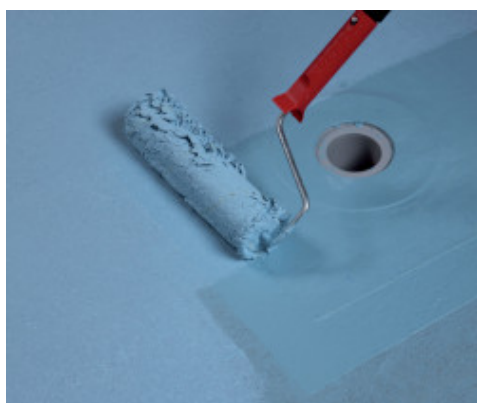
Application by roller of the second coat of Mapelastc AquaDefense Zero
