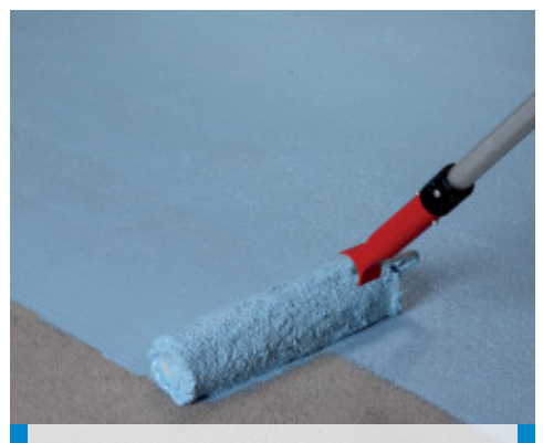
Application of the first coat of Mapelastc AquaDefense Zero on a screed
