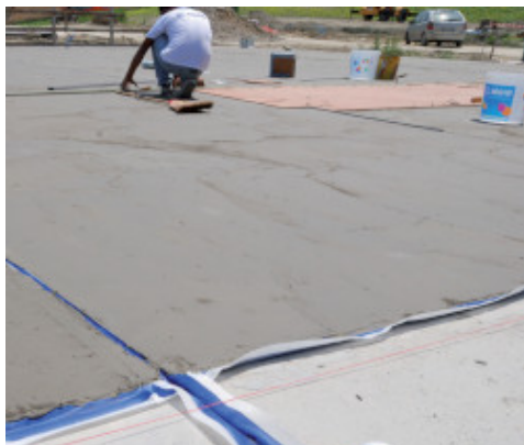
Waterproofing screeds with Mapelastic Zero and Mapeband
