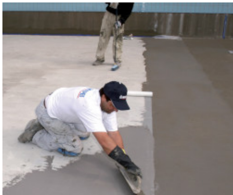
Waterproofing a swimming pool with Mapelastic Zero
