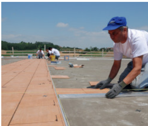
Installing ceramic tiles with Kerabond + Isolastic
