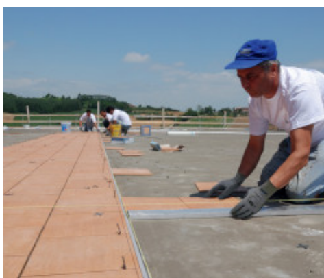
Laying ceramic tiles with Kerabond + Isolastic
