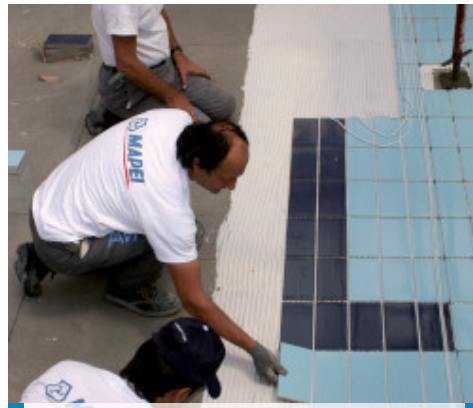
Application of ceramic coating on Mapelastic
