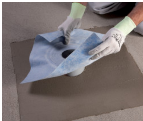
Application of Drain Vertical on Mapelastic
