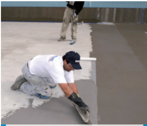
Waterproofing a swimming pool with Mapelastic
