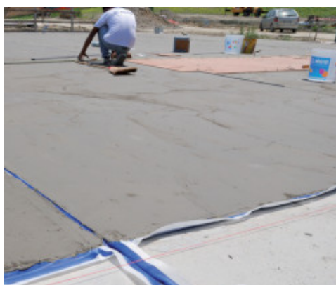
Waterproofing screeds with Mapelastic and Mapeband
