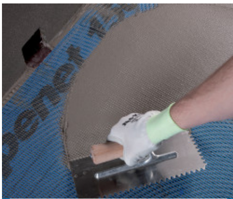
Application of Mapelastic on Mapenet 150
