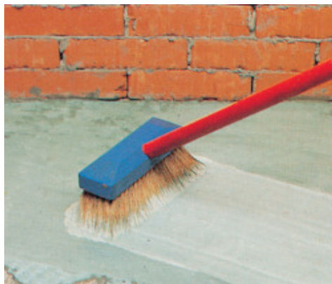
Application of cementitious grout with Planicrete Latex admix
