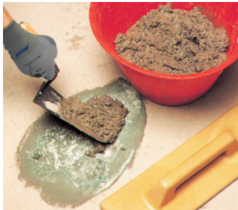
Floor patching: application of mortar
