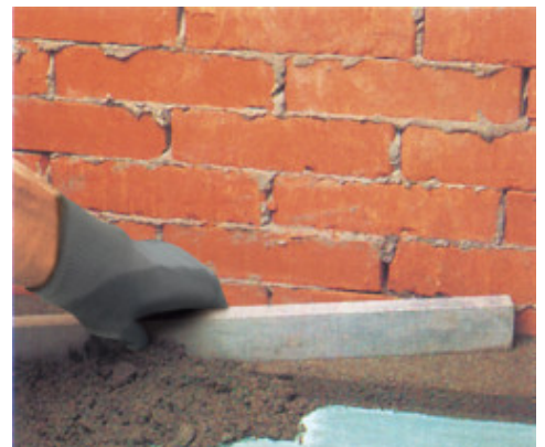
Application of cementitious screed with Planicrete Latex admix
