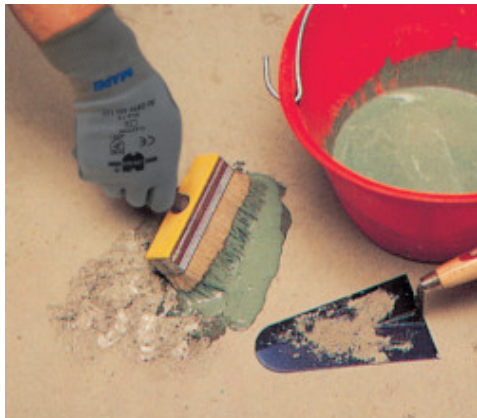
Floor patching: application of slurry
