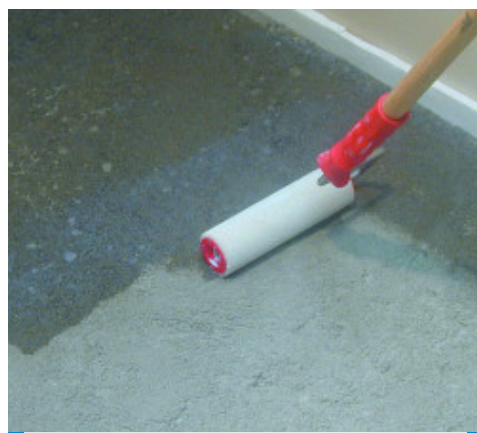
Applying Primer G with a roller
